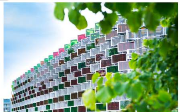
Figure 3: Semi-transparent BAPV in different colors on a parking house in Linköping in Sweden. Product is called Soltech Façade Semi-transparent. Photo: SolTech Energy.
