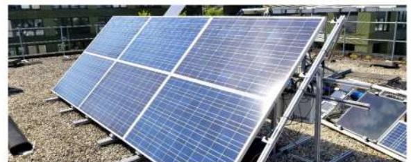
Figure 2: 6 pc-Si PV modules in series at GeePs rooftop under operation since Feb. 2019
