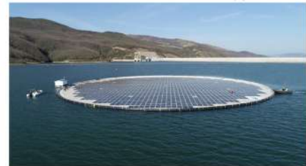
Figure 1: Floating unit of 500 kW p (Statkraft, 2021).
