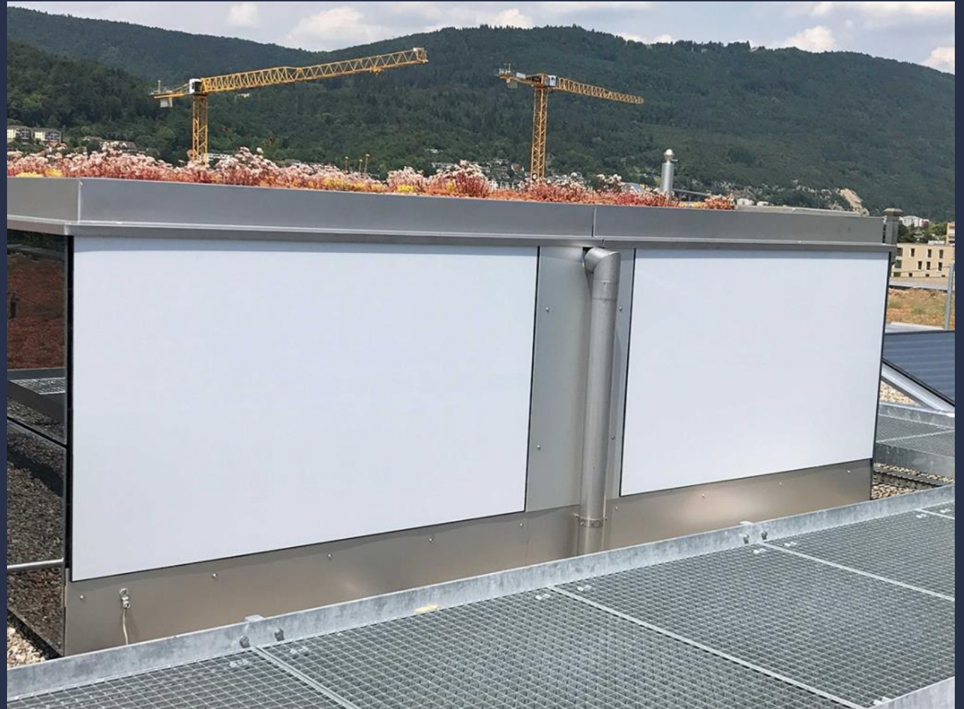
White PV panels, together with Solaxess
