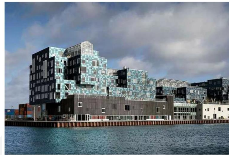
BIPV, International School of Copenhagen
