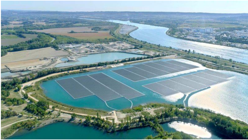
Floating PV plant, France
