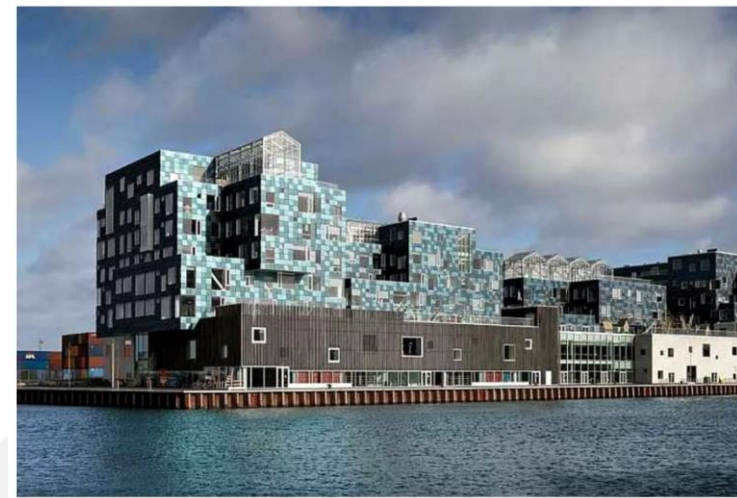
BIPV, International School of Copenhagen
