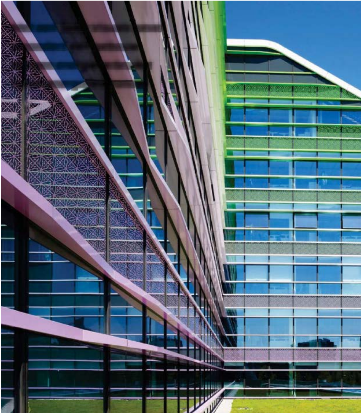
UNStudio Office retrofit design, colored PV in spandrel panels of a curtain wall
