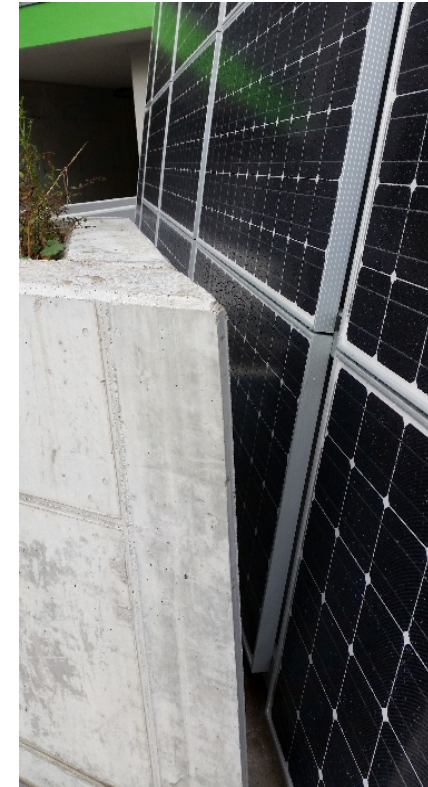
Shading problems due to nearby object / bad planning
